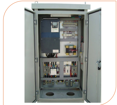
Hoist control panel box
